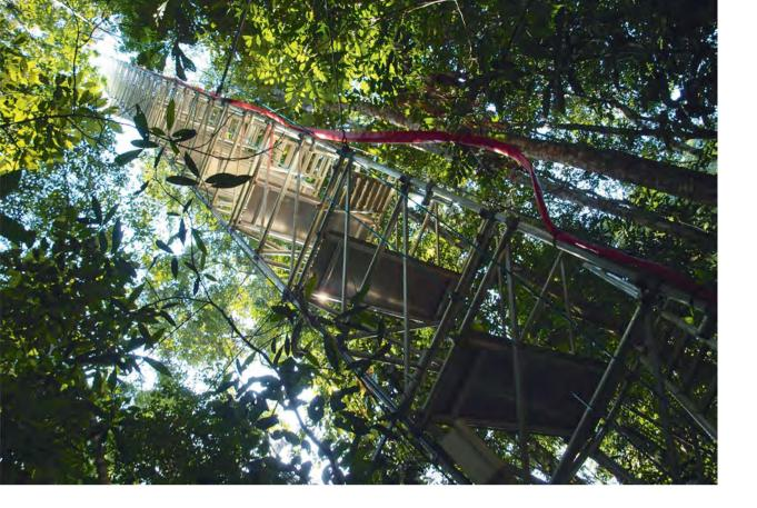
mountain hike up to the tower. In reality, this is nothing more than an open staircase held in place by steel cables, and it takes the scientist around three quarters of an hour to climb the 325 meters to the top.
