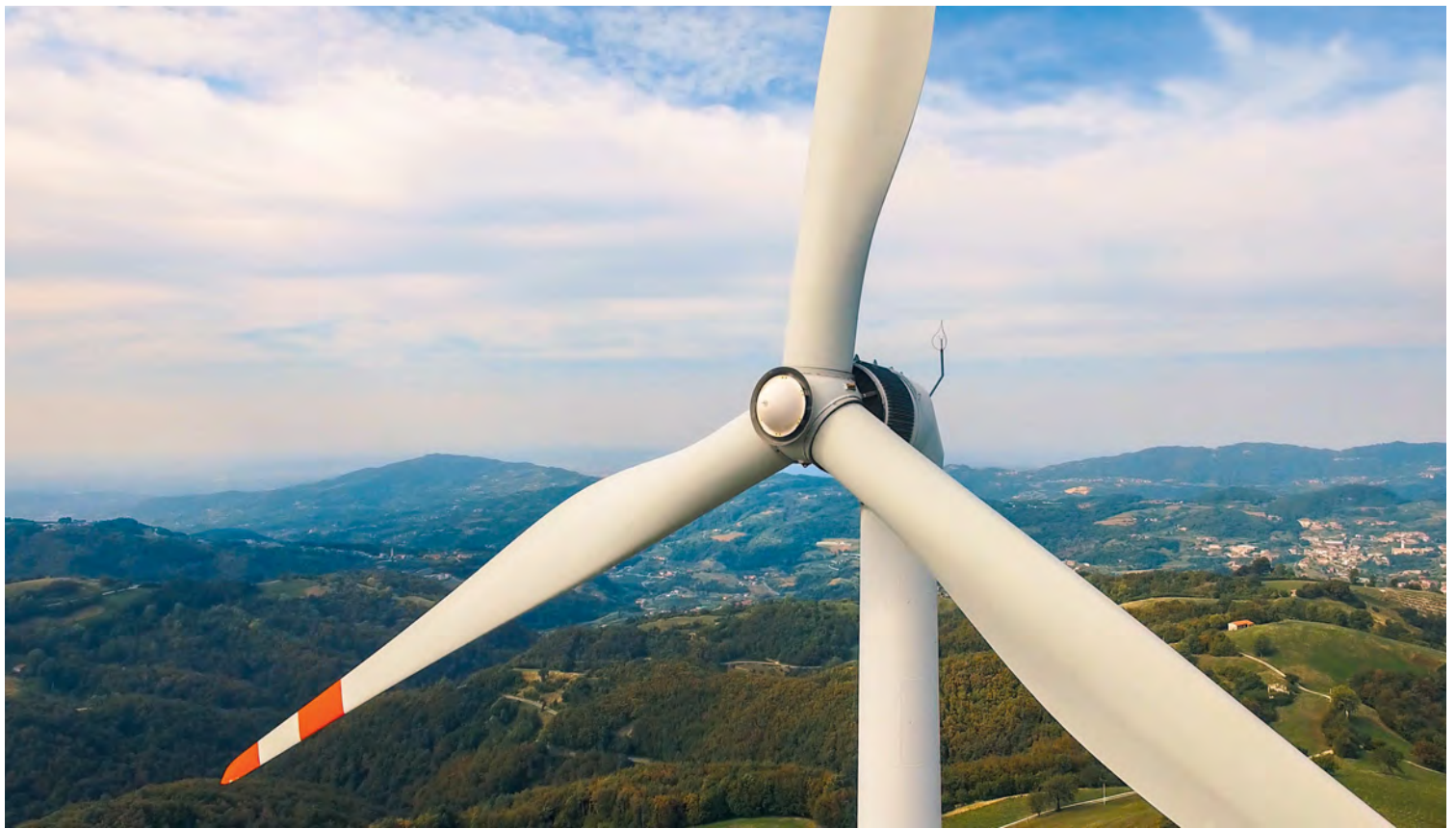
The power of mathematics: Holger Kantz's team has found a way to use measurements of wind strength to predict particularly strong gusts at short notice. Wind turbines can then be protected by altering their rotor blades' angle of attack.
