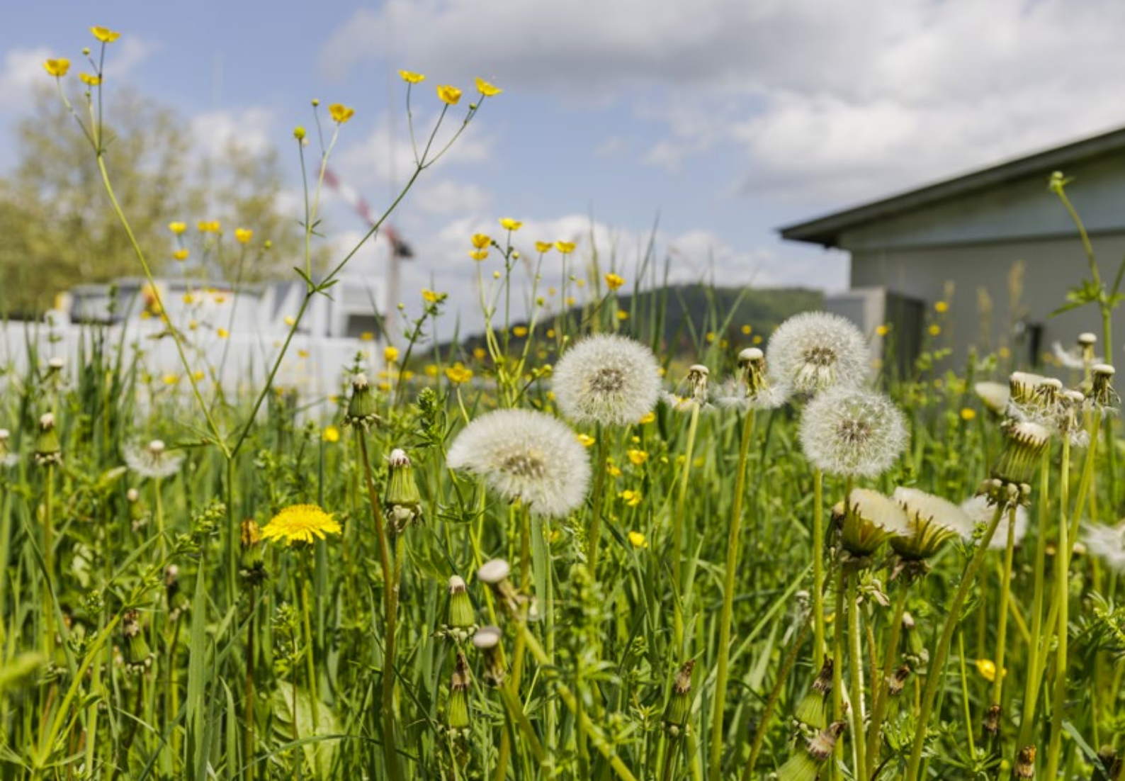
Green roof of the MPI for the Study of Crime, Security and Law, Freiburg
