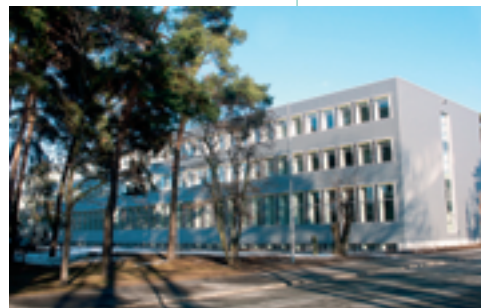
The modernized Max Planck Research Group building on the Siemens research campus in Erlangen.
