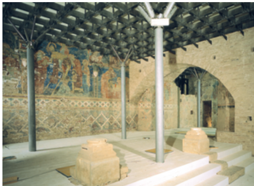
A view of the exposed under-church with its decorative frescoes dating from around 1280. The choir of the church above is supported by a modern system of stanchions.
