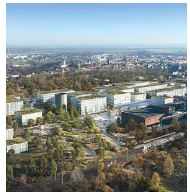
PHOTO: HDR GERMANY
