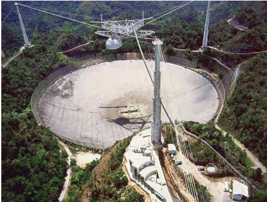
Left A satellite dish surrounded by nature: The Arecibo radio telescope in Puerto Rico has a diameter of 305 meters and listens for pulsar signals. Einstein@Home can detect them, thus transforming home PCs, smartphones and tablets into valuable tools for science.
